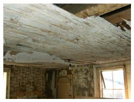
The house was occupied for 250 years by DuBois descendants, with little maintenance during the last 100 years, so it is not surprising that the house had become derelict and in danger of falling down. The tin roof leaked, shingles were missing causing massive water damage, and plaster and lath ceilings were falling down. Second floor supports had rotted and started to fall and support posts in the cellar were sinking into the ground; 250 years of history were being consumed by neglect.
