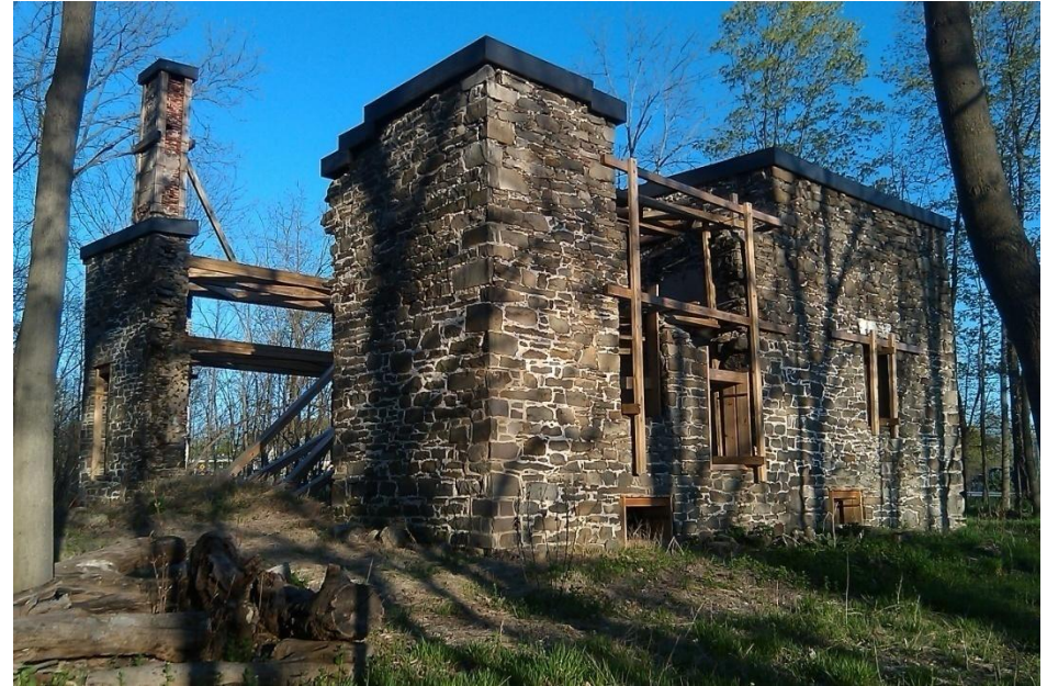
Northeast corner (facing SW)
